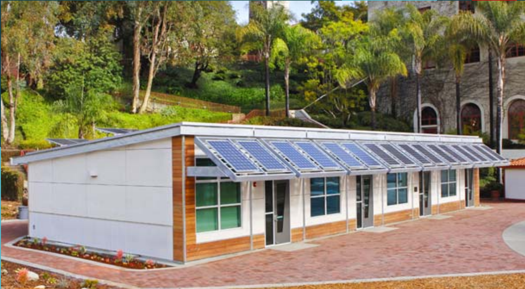
American Modular Systems Gen 7 Classrooms School
