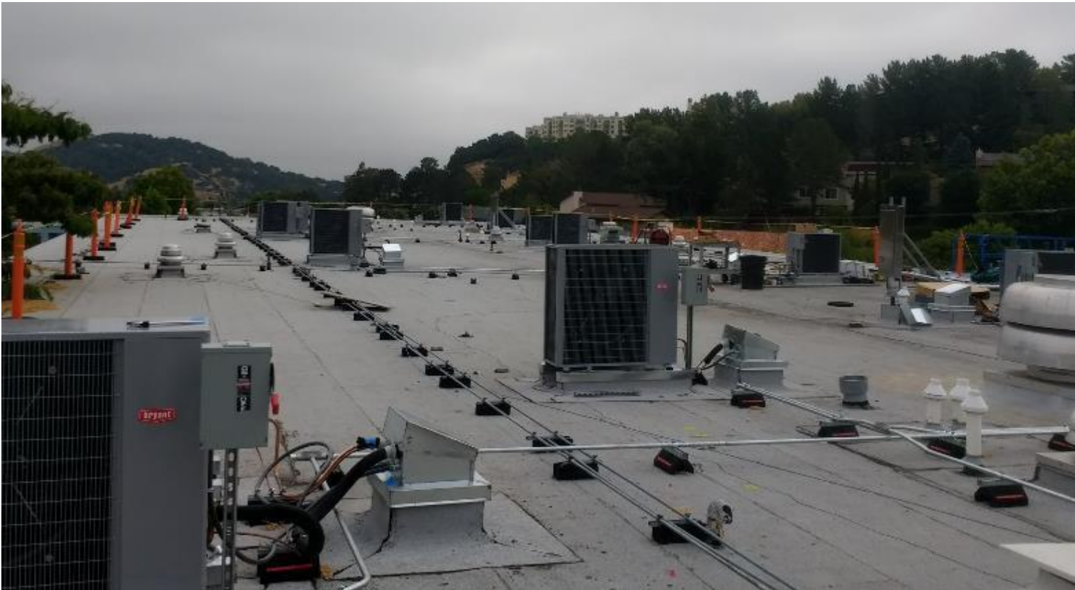
Terra Linda HVAC Project
