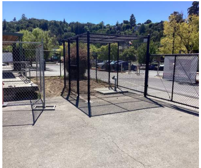
PG&E gas meter chain-link fence enclosure
