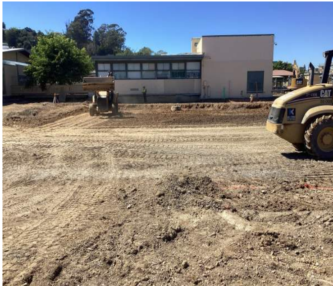
Rough grading work on-going w/ heavy equipment
