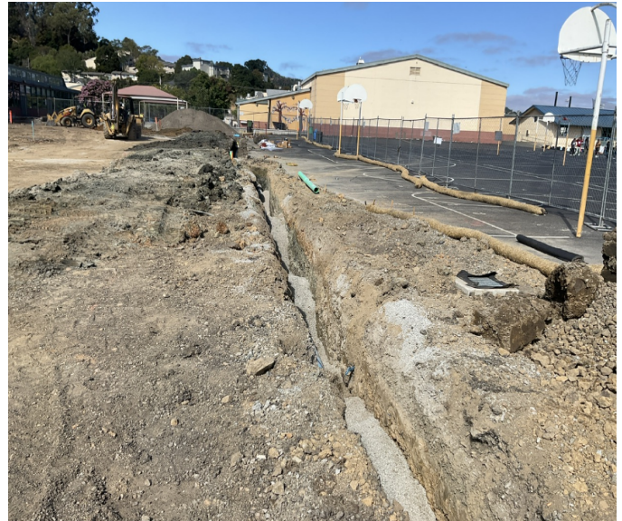
Fire Water pipe install at trenches prepping for backfill and compaction
