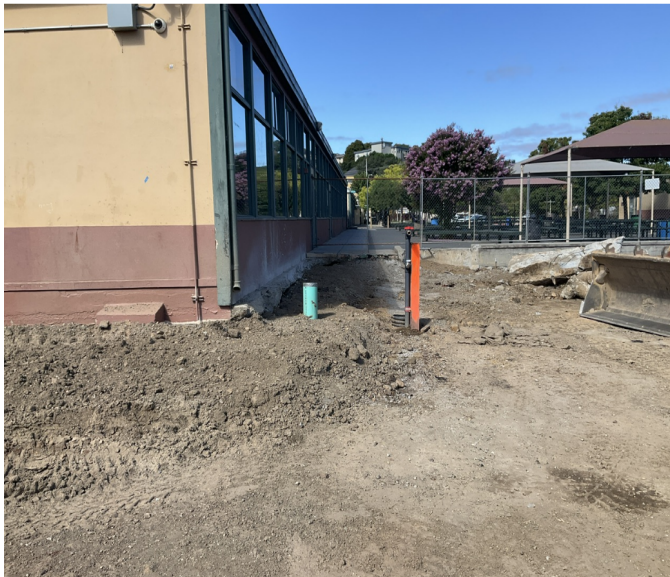
New fire water shut off valve stand pipe during grading work
