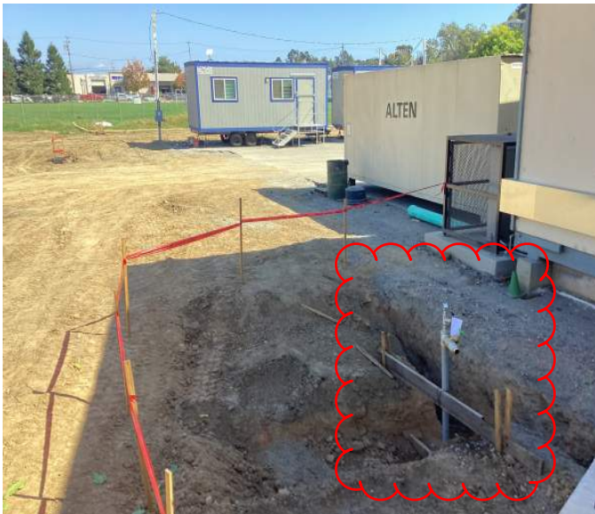
Underground domestic water chlorination stub up POC #1
