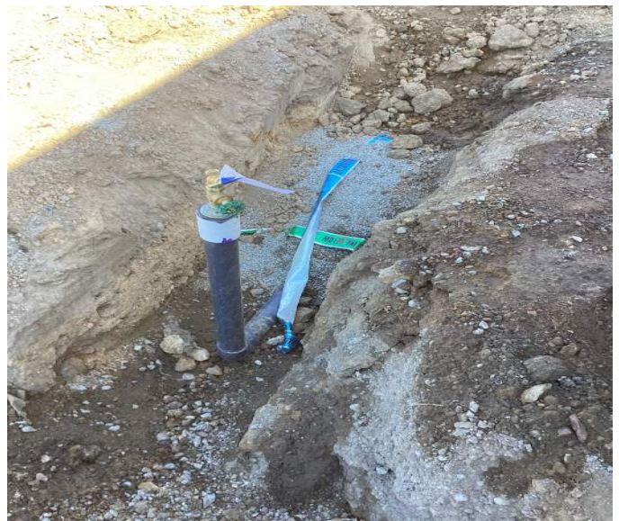
Underground domestic water chlorination stub up POC #2
