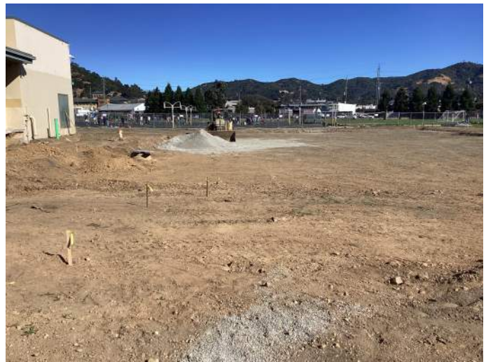
Site surevey and staking for the SS line
