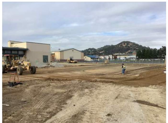
MPR pad lime treated, mixed, rolled, and compaction completed
