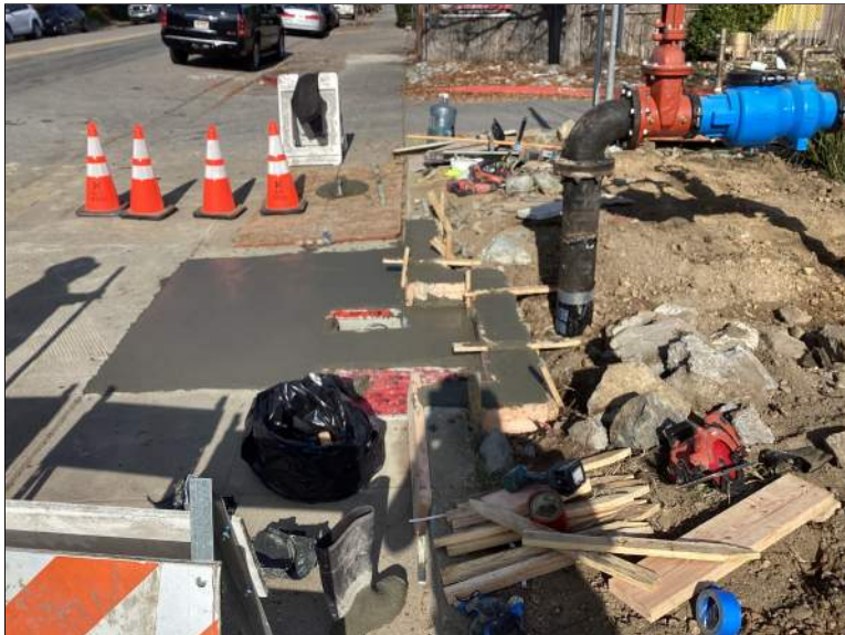
Front of campus MMWD Backflow Assembly install and concrete sidewalk pour
