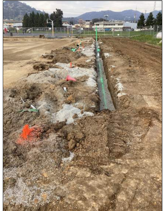
Sanitary Sewer Line pothole, line tie-in, and backfill on site
