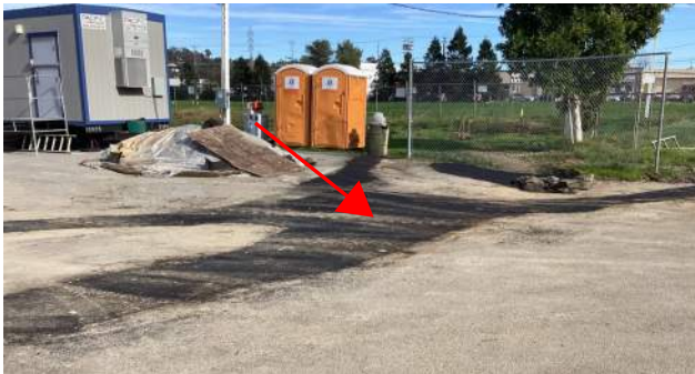
Temporary construction access road install - 80% complete shown below
