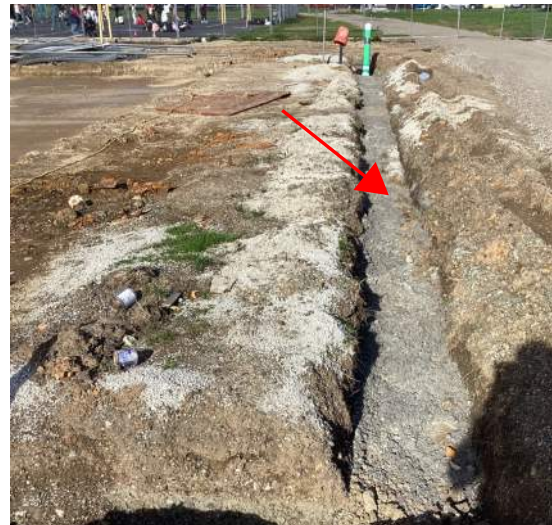
Sanitary Sewer trench with concrete cap poured
