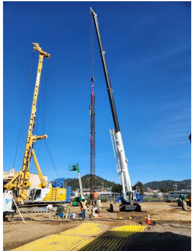
Rebar cage being placed in pier foundation hole
