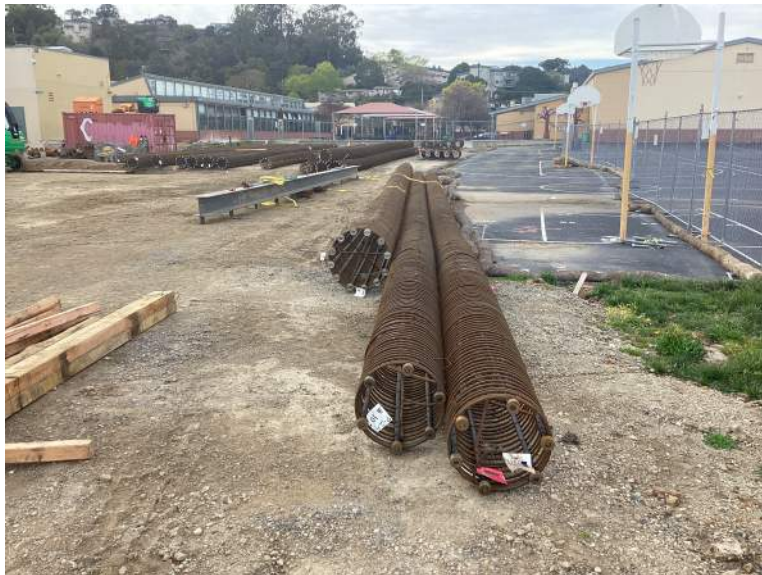
Rebar cage material delivered
