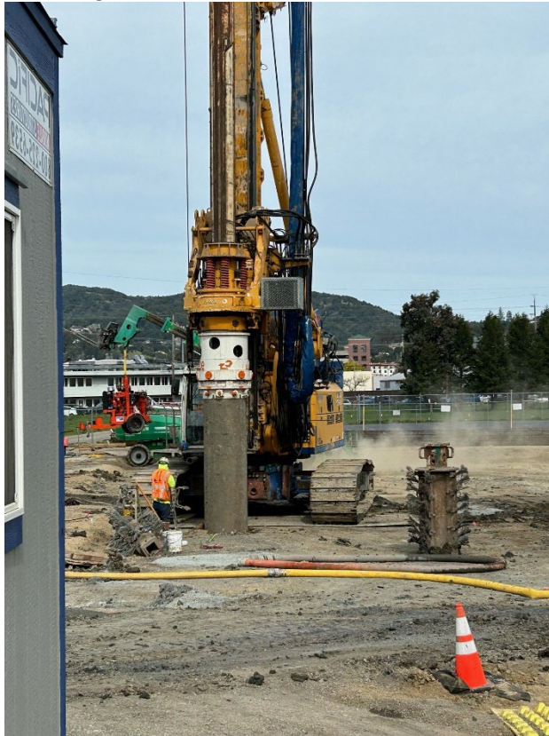
Pier Drilling for MPR Foundation
