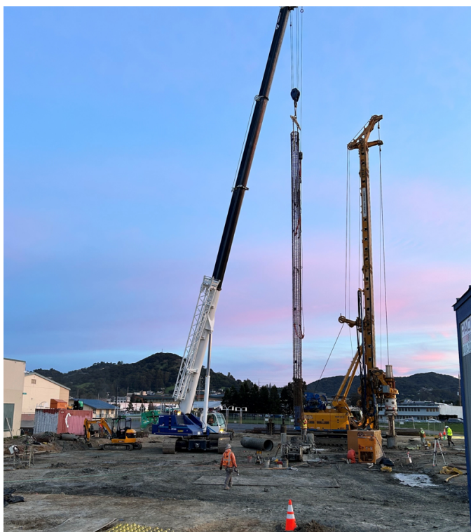
Rebar cage placement at pier foundation
