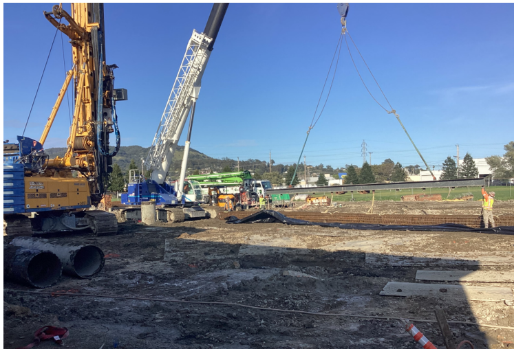
Rebar cage staging for pier foundations
