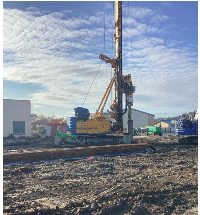
Drilling of foundation pier completion at end of day
