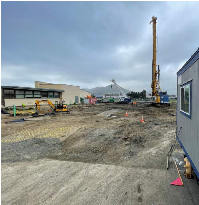
Core drilling of the 24" Diameter foundation piers
