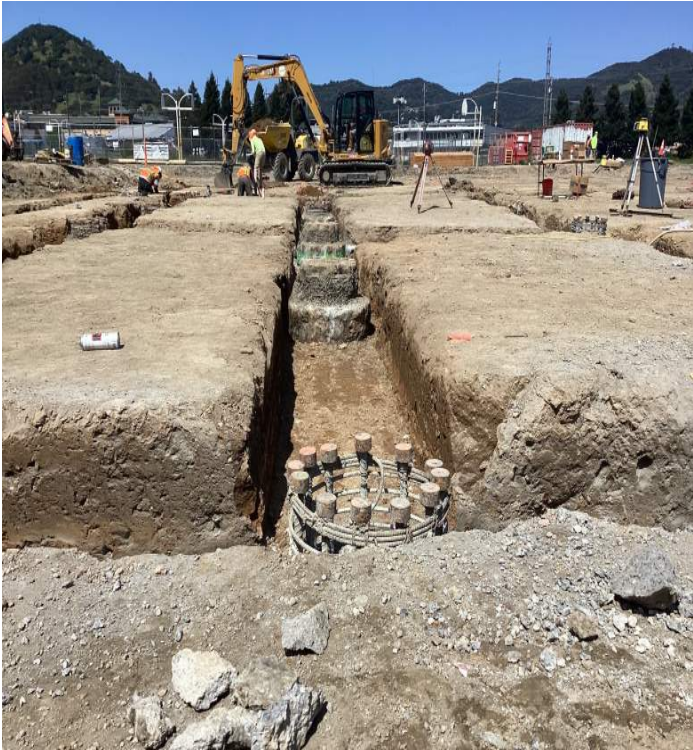
MPR foundation grade beam excavation
