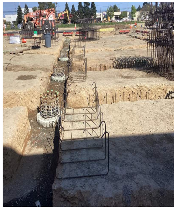
Grade beam steel shake out and install at trenches
