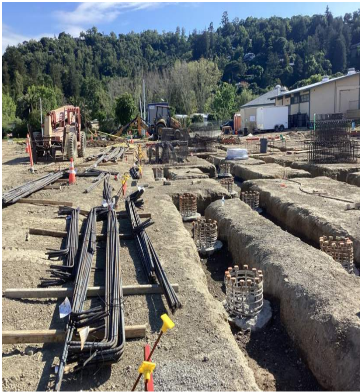
Rebar & Grade beam steel material delivered onsite
