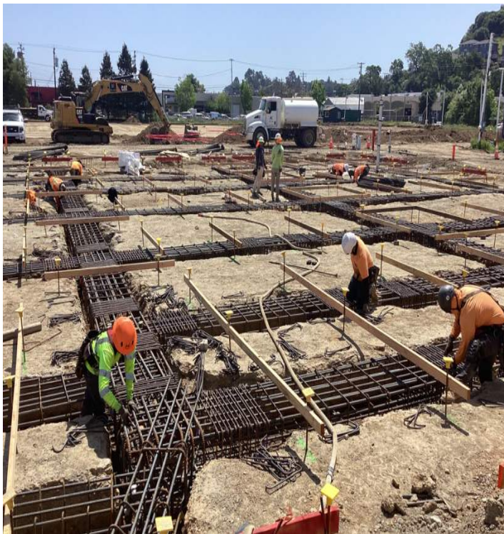
MPR - Grade beam rebar & formwork installation
