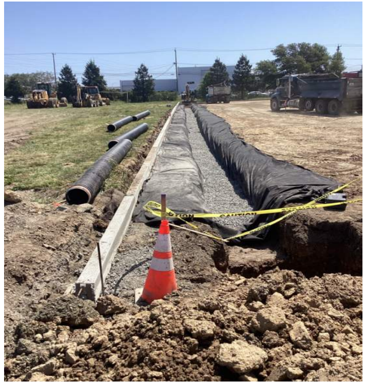
FIELD - Perforated storm drain pipe placement in trench with bed rock backfill
