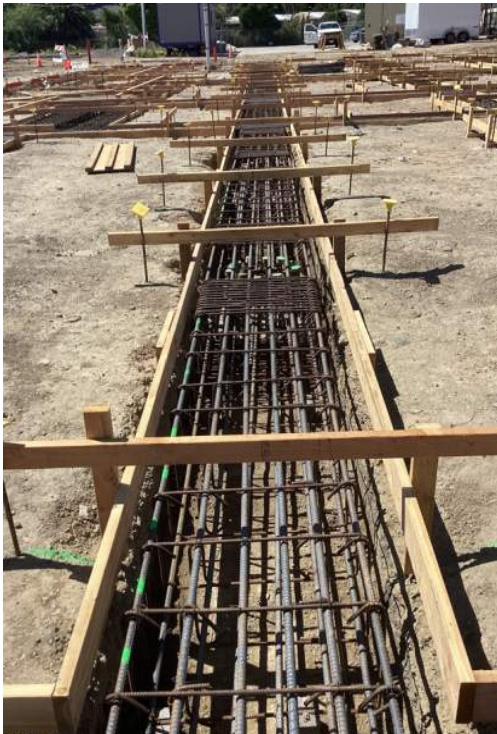
MPR - Rebar & formwork installation continued
