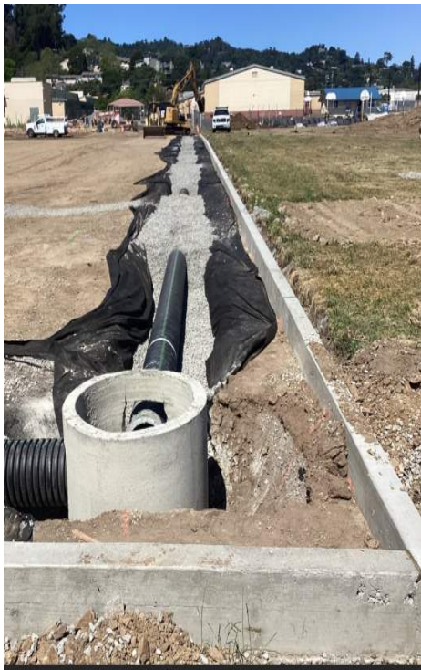
FIELD - Perforated pipe installed and covered with base rock. Poured concrete curbs
