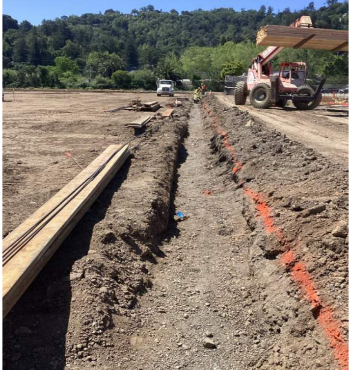
FIELD - Trenching and digging of new concrete gutters and curbs around the field
