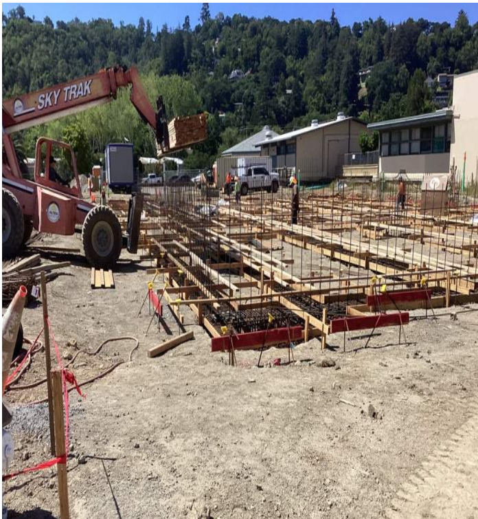
MPR - Rebar and form-work install in preparation for concrete pour
