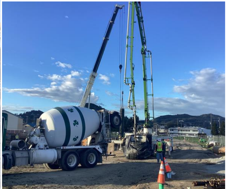
Concrete/slurry pump truck filling drilled piers.
