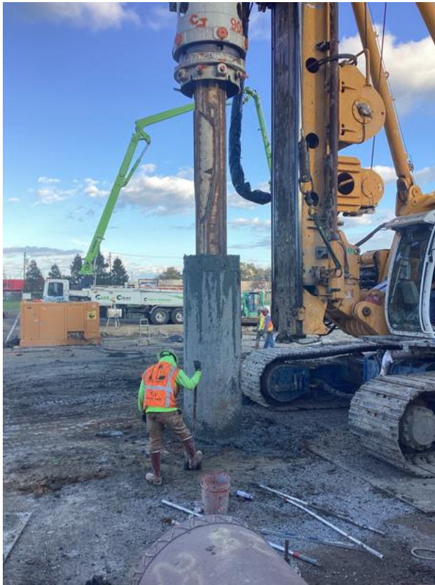
Pier drilling on-going.
