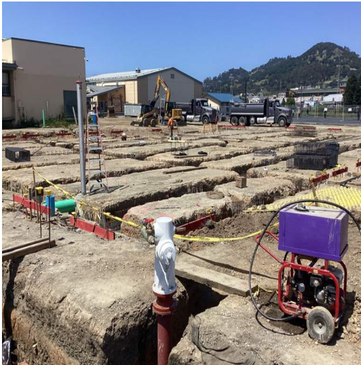
MPR - Grade beam rebar install @ 8" Fire Riser
