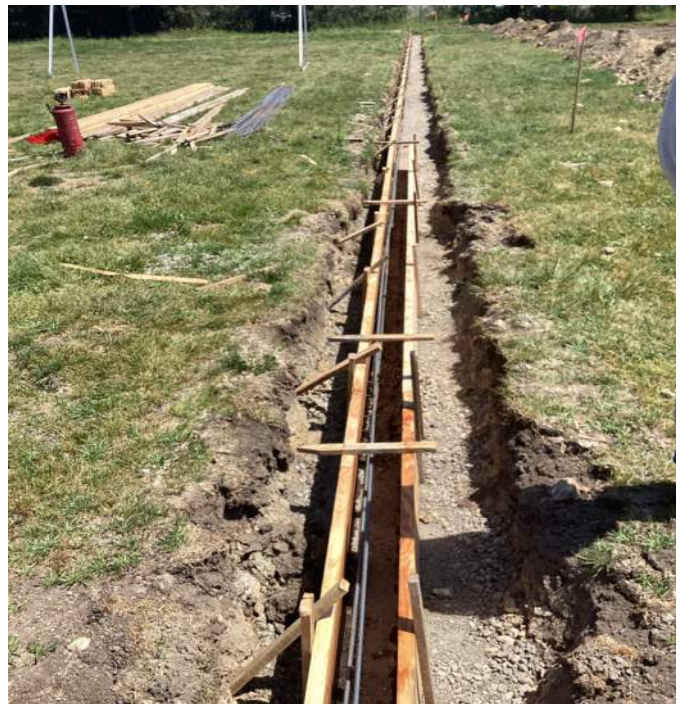
FIELD - Mo-band trench framing and rebar install
